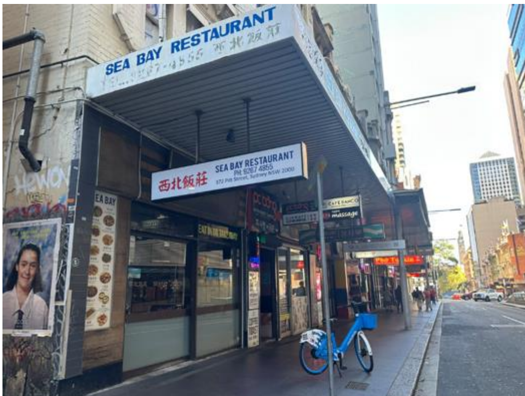
Figure 5: Site viewed from Pitt Street footpath facing south towards Goulburn Street
