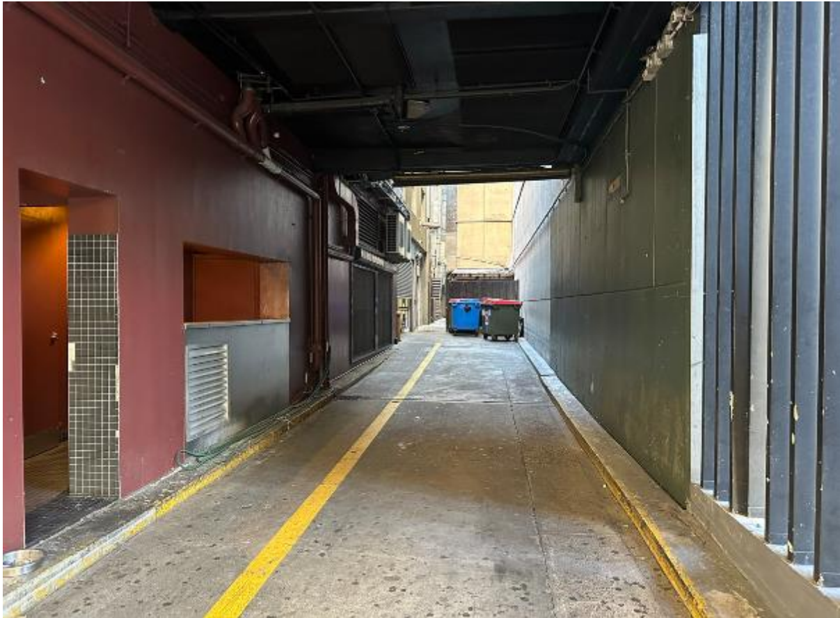
Figure 11: View of restricted vehicular right of way from Goulburn Street, through Civic hotel facing north (looking back towards the rear of subject site)
