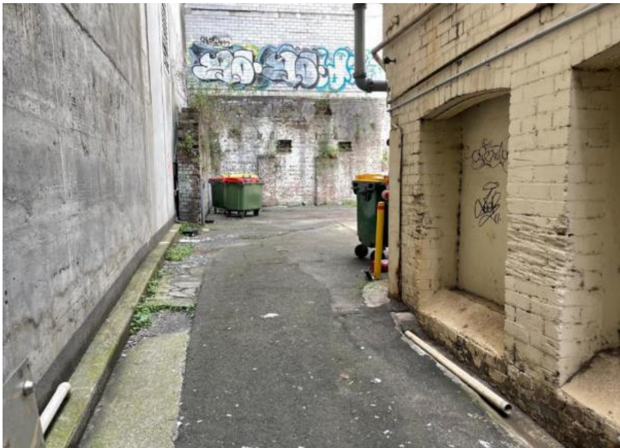
Figure 7: Carruthers Place rear facing east
