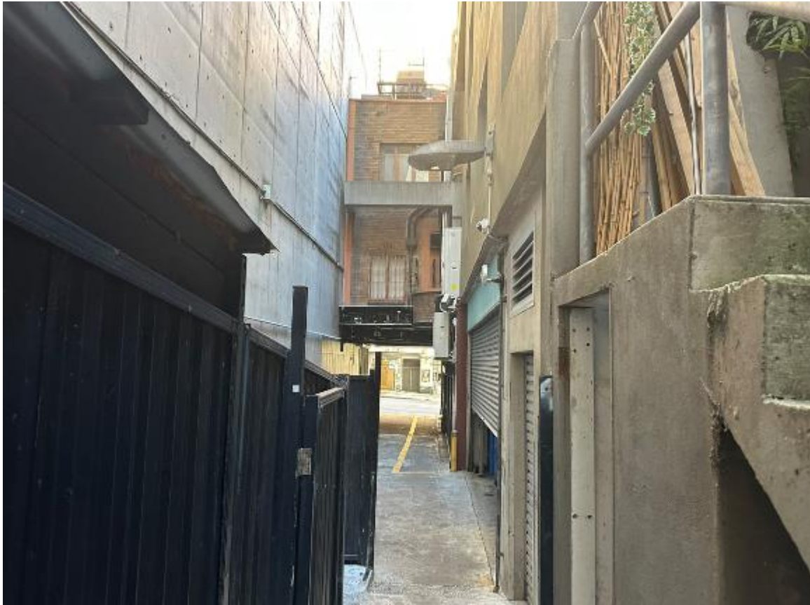
Figure 10: Rear site interface, viewed from behind 382-382A Pitt Street looking to restricted vehicular right of way to Goulburn Street
